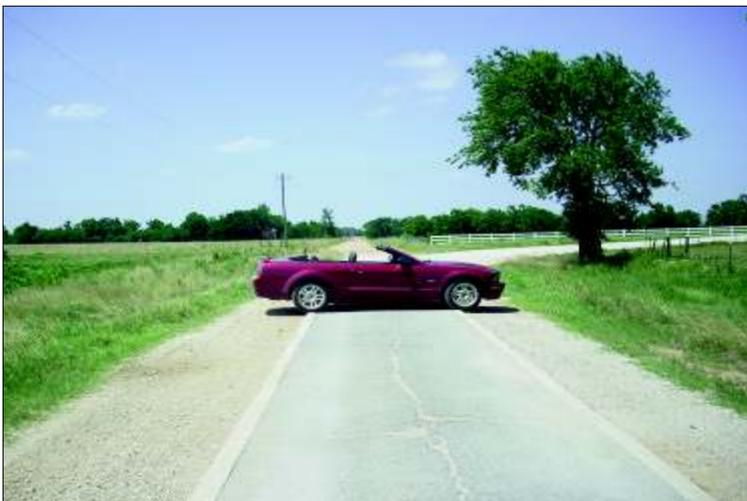
*This photo was taken on the 9 foot ribbon highway on a section between Afton and Narcissa, OK. The wheelbase of the Mustang is 107 inches.*
